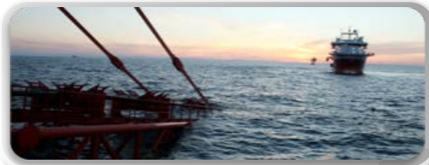
Offshore Pipelines and Platforms Installation
