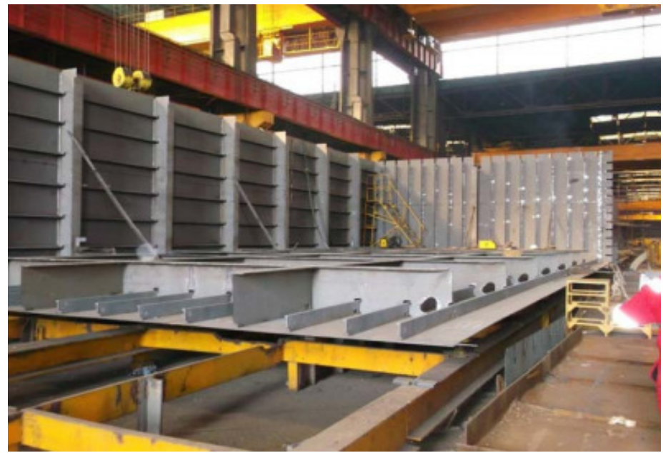
Construction of Shallow Water Barge
