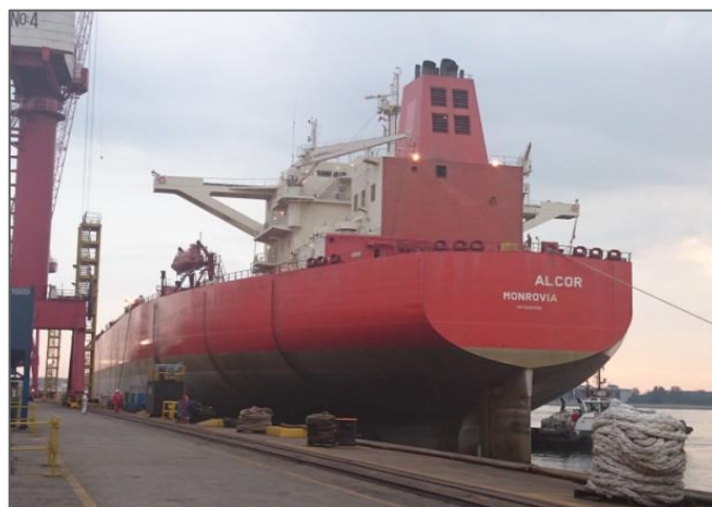
Conversion work on-going on Kraken FPSO
