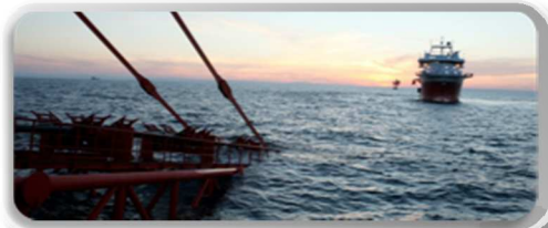
Offshore Pipelines and Platforms Installation
