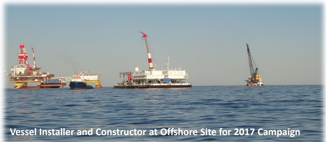
Vessel Installer- Bridge Installation
